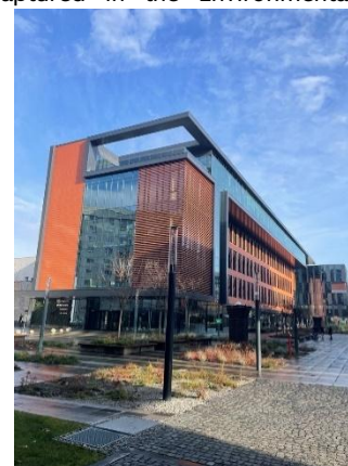
BREEAM certified Cluj, Romania office building
